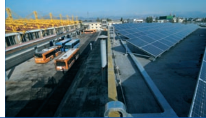
The photovoltaic panels are installed on the depot roof in Naples, in Southern Italy, where they catch the most sunlight.
